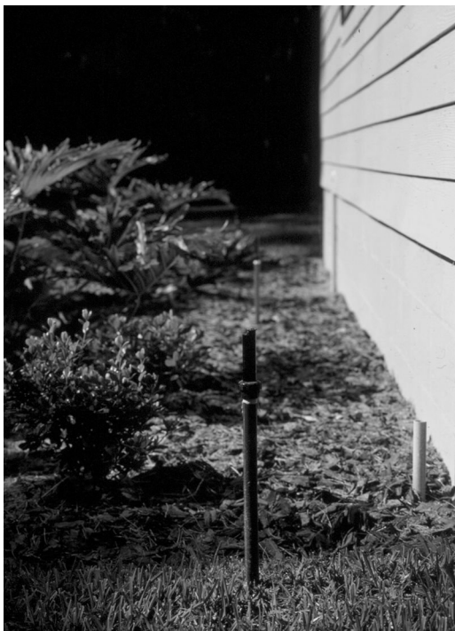
△ FIGURE A.17.1.8.1(b) Use of Low Volume Sprinklers in Organic Material. (Courtesy of Firewise Communities Program. Photo by G. Johnston.) [1140:Figure A.A.24.3.4.1(b)]
