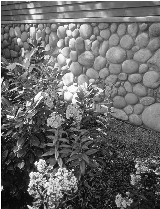
△ FIGURE A.17.1.8.1(a) Foundation Planting and Landscaping. (Courtesy of Firewise Communities Program. Photo by K. Clineff.) [1140:Figure A.24.3.4.1(a)]
