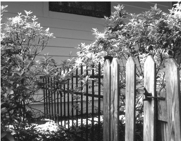
▲ FIGURE A.17.1.8.3(b) Transition Fence Separates Combustible Fence from Structure. (Courtesy of Firewise Communities Program. Photo by G. Johnston.) [1140:Figure A.24.3.4.3(b)]
