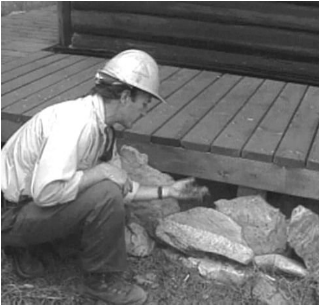
▲ FIGURE A.17.1.8.3(a) Leaf Litter and Needles Collect in Small Spaces. (Courtesy of Firewise Communities Program.) [1140:Figure A.24.3.4.3(a)]
